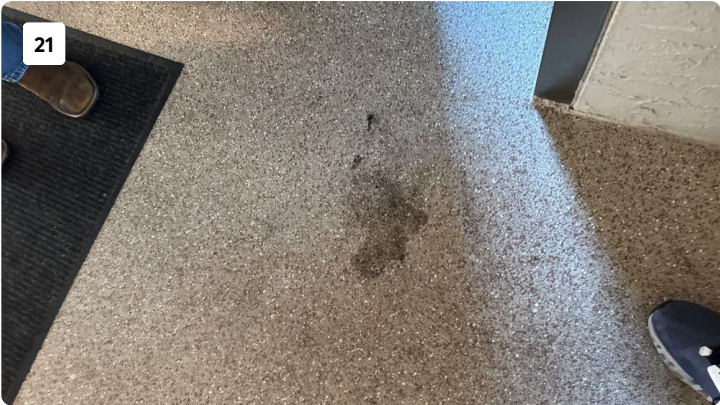
walk way protection to be installed.
