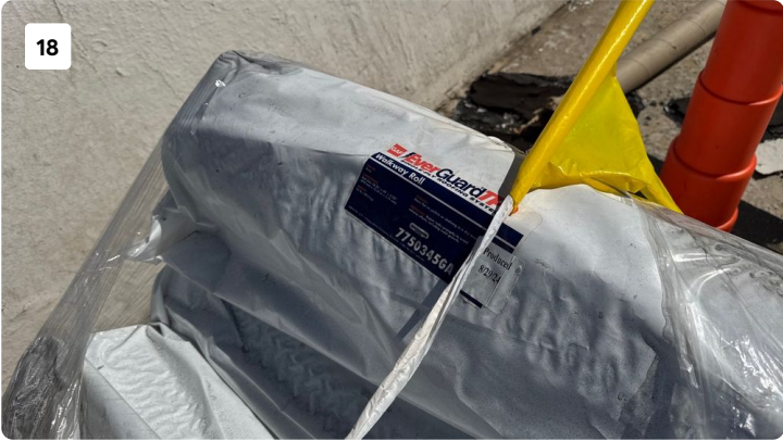
proper material are loaded on the project per the specifications.
