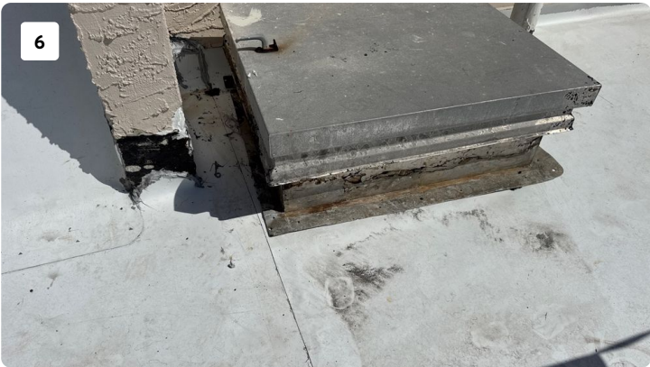
the old curb was removed and is stored for re-installation.
