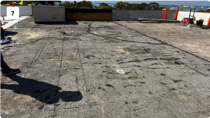
lightweight concrete looks to be in good condition.
