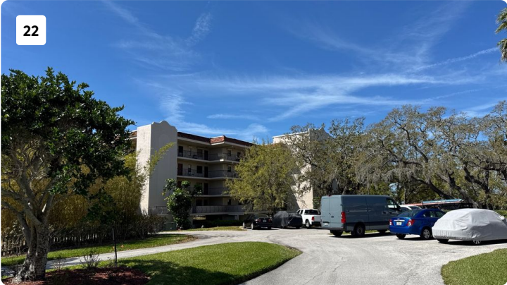
Front of Bldg #2
